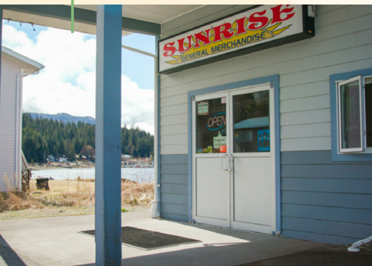
Gizuá Market before renovations. Photo: yáqwa Development Corporation
